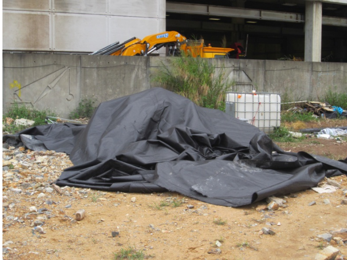
Photo 1 – Impermeable sheets were observed to have been placed on the stockpiles of excavated soils and rocks that were not in use.
