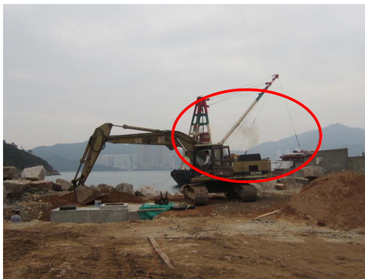
Photo 3 – Dark smoke was seen rising from the crane truck used to backfill the excavated rocks and soils.
